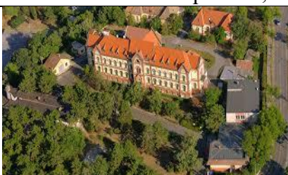
Nyár Street campus site, Pécs
