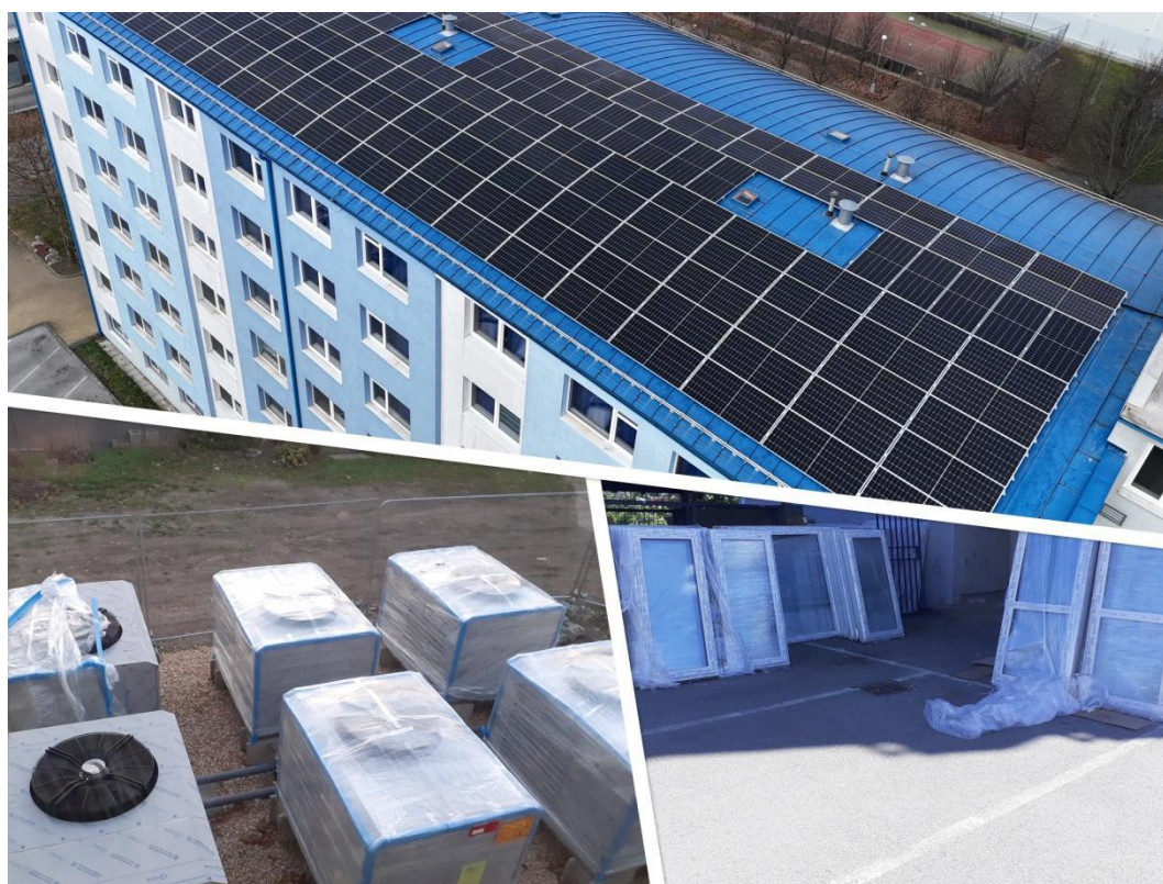
Picture 8: Solutions within accommodations
